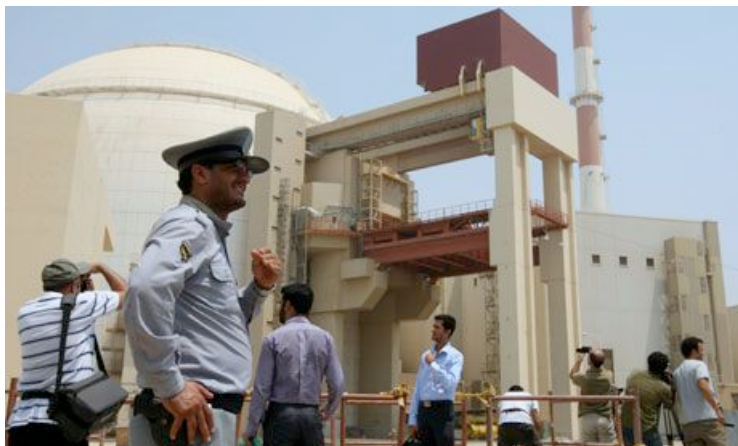
Iran's Bushehr nuclear power plant. Photograph: Atta
