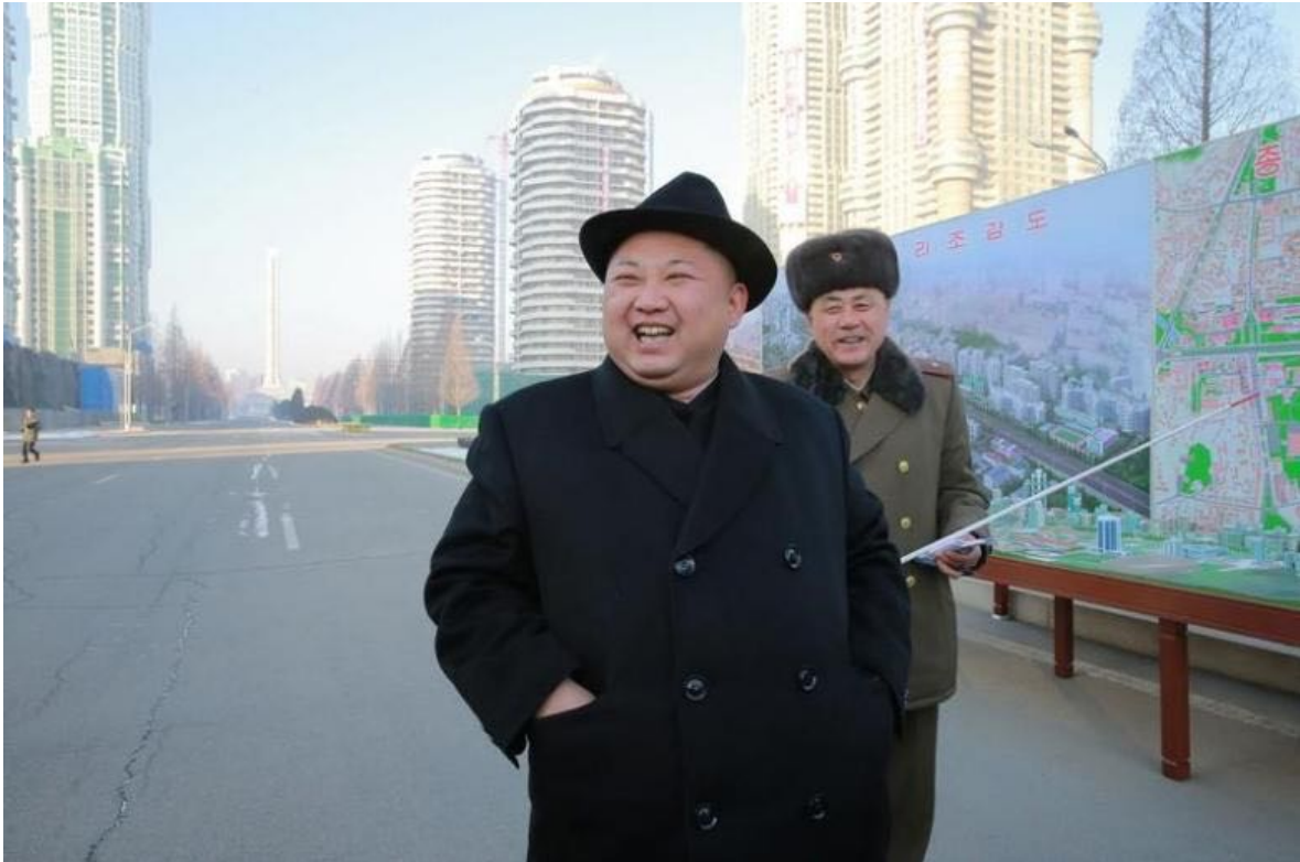
North Korean leader Kim Jong Un inspects the construction site of Ryomyong Street, in this undated photo released by North Korea's Korean Central News Agency (KCNA) on January 26, 2017. KCNA via REUTERS
