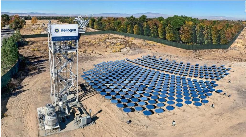
Heliogen, backed by Bill Gates, has achieved a breakthrough that could allow cement makers to transition away from fossil fuels. The company uses artificial intelligence and an array of mirrors to create vast amounts of heat, essentially harnessing the power of the sun.
