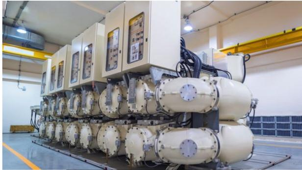
Gas-insulated, high-voltage switchgear almost always uses SF6
