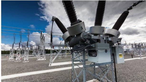
Electrical switchgear the world over often uses SF6 to prevent fires
