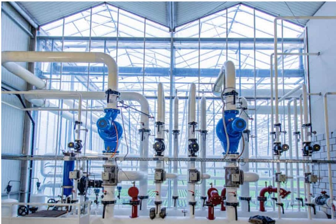
Gauges, valves and pipes for water, heating and CO<sub>2</sub> at the Gebr Meier greenhouse in Hinwil outside Zurich. The heating and the CO<sub>2</sub> is sourced from the local waste incinerator, where the CO<sub>2</sub> is collected by the Swiss company Climeworks. Photograph: Orjan Ellingvag/Alamy
