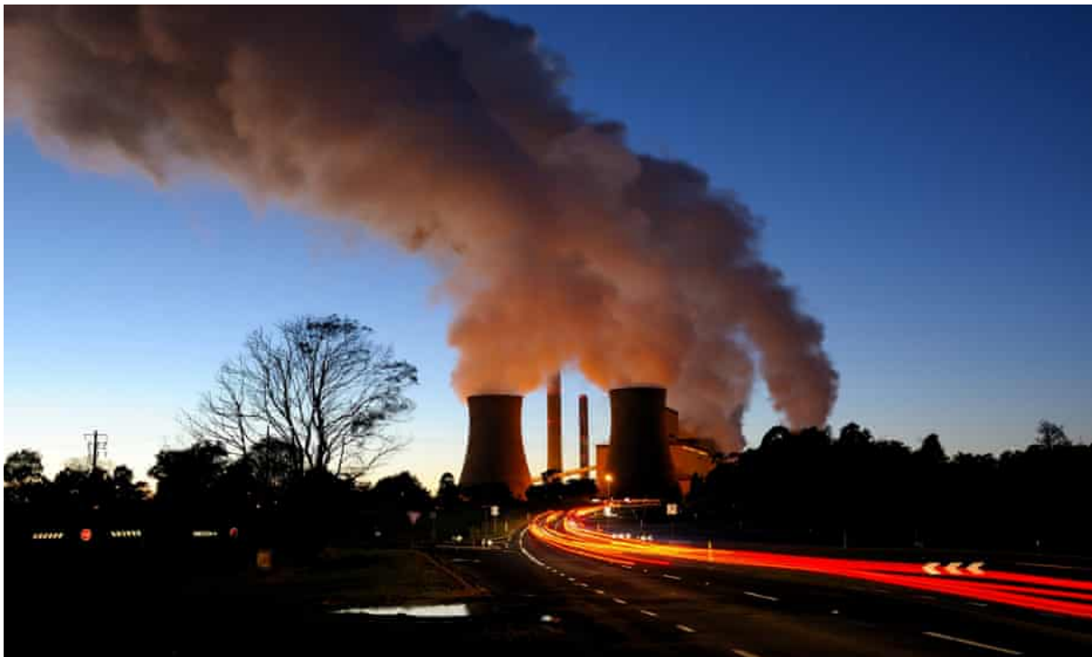
AGL, the country’s biggest greenhouse gas emitter, has announced it will build a large-scale battery next to its Loy Yang A coal plant in Gippsland. It is the third major battery announcement in two weeks. Photograph: David Gray/Getty Images
