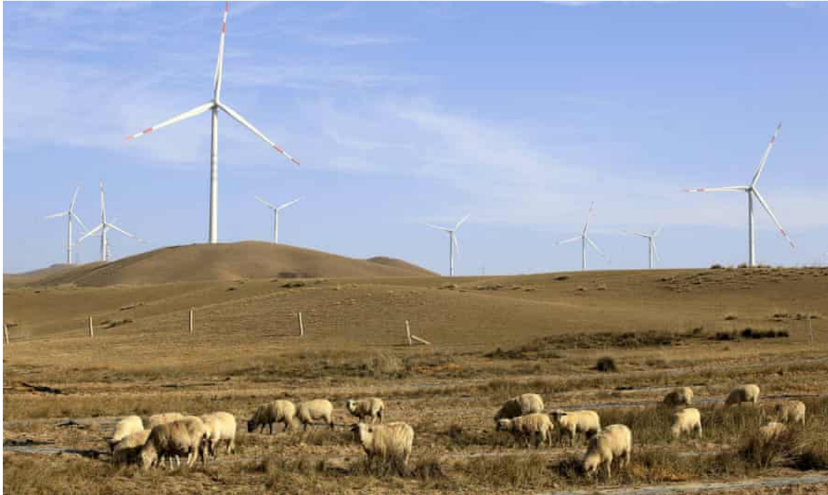
Wind turbines in Gansu, Wuwei, China, pictured in November 2020. Photograph: Rex/Shutterstock
