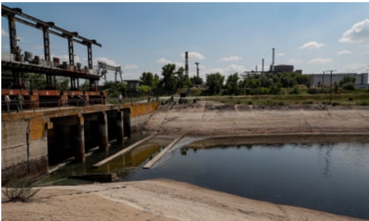
Water levels fell at the Kakhovka reservoir after the destruction of the Nova Kakhovka dam, the IAEA reported in June 2023. The Zaporizhzhia power station draws water from the reservoir for cooling. Photograph: Sergei Ilnitsky/EPA
