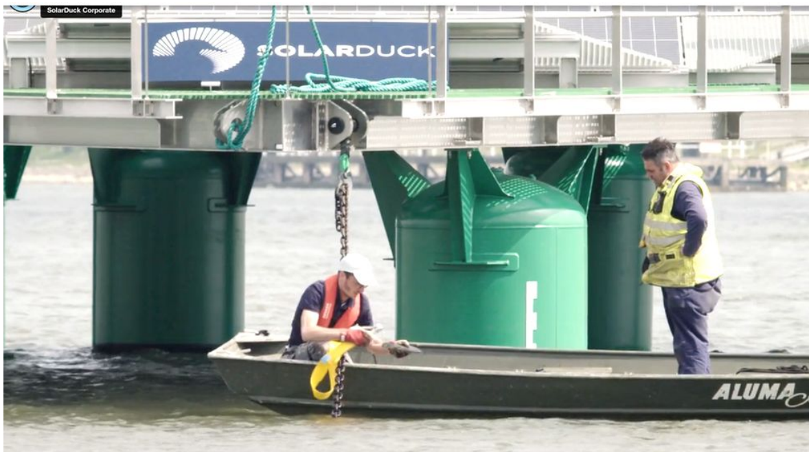
SolarDuck puts solar panels on a raised platform to protect them
