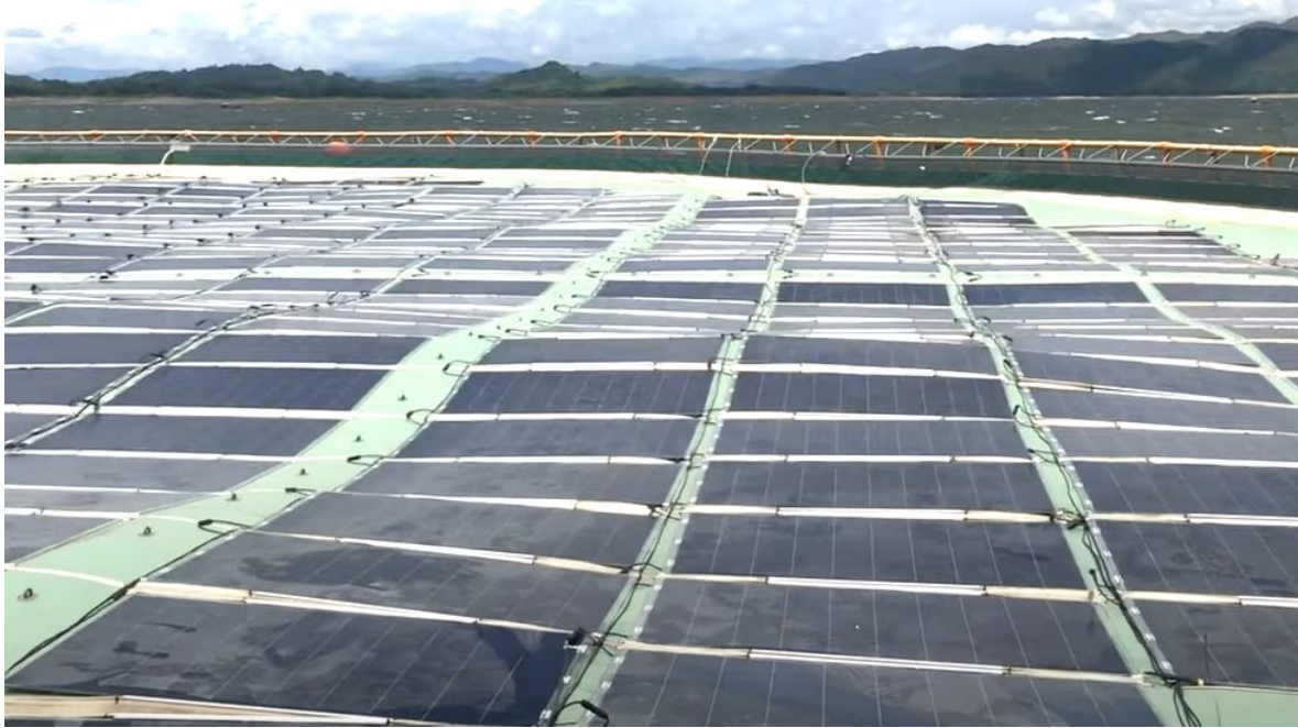
The base of the Ocean Solar plant flexes as waves move underneath it
