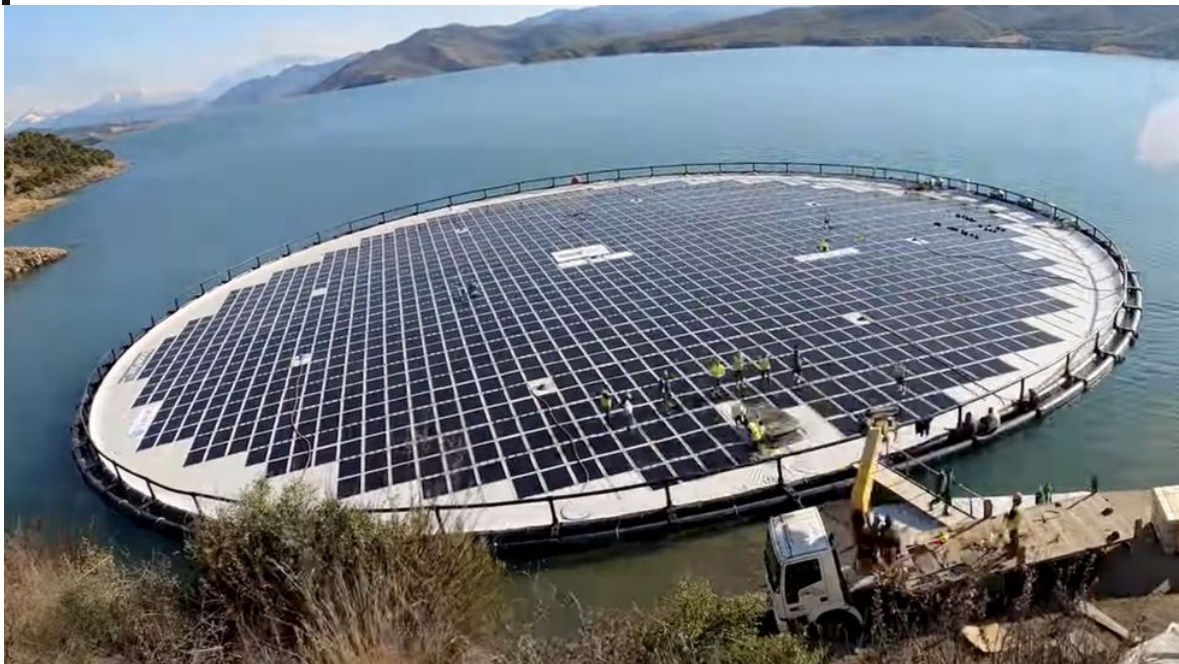
Ocean Sun solar panels sit on a flexible floating pad
